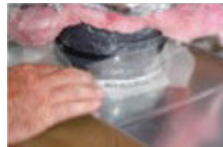
Install tie strap and apply fiberglass mesh tape.
